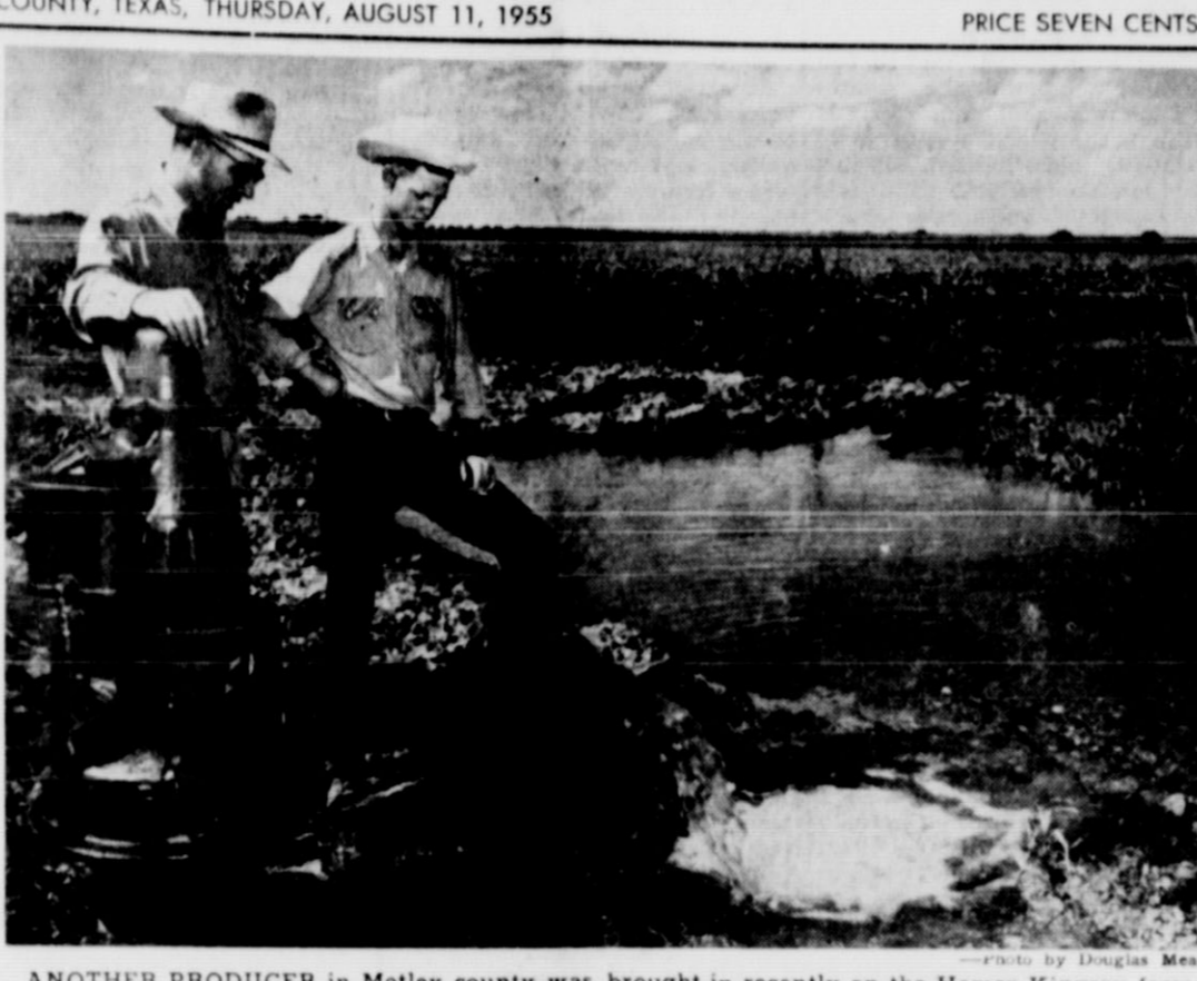
ANOTHER PRODUCER in Motley county was brought in recently on the Homer Kingery farm in the Darden Canyon community. In the above photo Ed Jameson, left, the driller, and his nephew, Roger Kingery, watch the test pump lift 400 GPM of clear, pure water from the 200-foot well. The well is rated as a good "five-inch" producer, although the test equipment is six-inch. Estimates are that sufficient water is available to irrigate 80 acres without any rainfall and approximately 125 acres with moderate rainfall. Constant development of irrigation in the county is causing land-owners to seek profitable water sands beneath fields long devoted to dry land farming. The above well is approximately 11 miles southwest of Matador.
