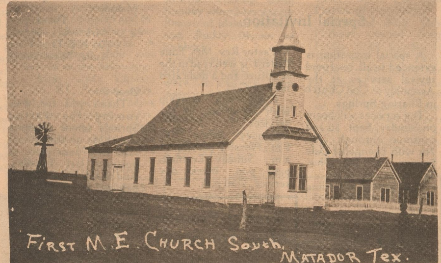
MATADOR'S FIRST CHURCH --For several years the only house of worship in Matador, the first Methodist church building was built in 1900 under supervision of T. N. Edmondson, with the Rev. C. A. Clark as pastor. The frame structure was about 30x50 feet and faced east, near the same location that the new building occupies. In above picture, the parsonage is shown at the right, but was later moved to another location.
