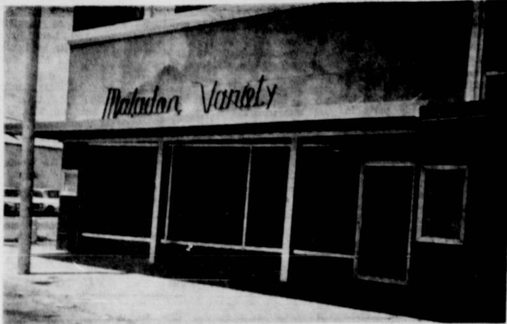
NEW LOOK in Matador is the Matador Variety front on the Masonic Building which was completed in the spring. The improvement has changed the appearance of the corner and greatly benefited merchandise display in the store. Glass used in the new front is shaded to prevent sun damage to merchandise. —Tribune photo and engraving
