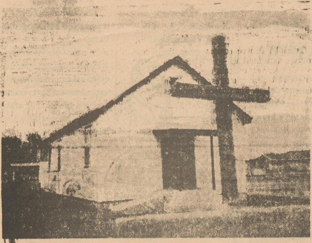
'TRAVELING' CHURCH — A little, white frame mission church building that has served at Rotan, Jayton, and Spur and which was hauled to Turkey recently, will be dedicated today as the new St. Elizabeth Ann Seton Mission Church.
