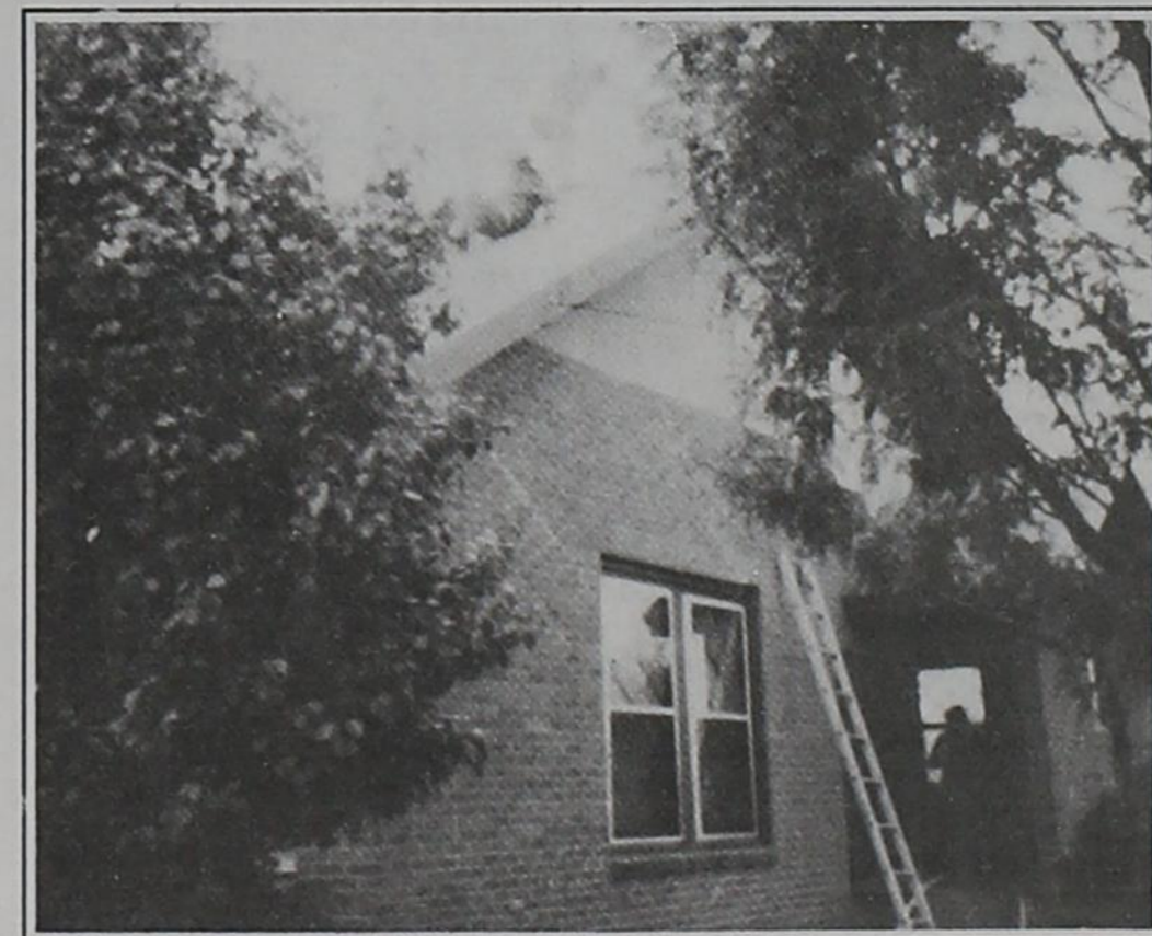
FIRE DAMAGES HOME — The home of Brent and Teresa Whitaker was damaged by fire last Thursday evening. Although it's hard to see in this picture, there are two firemen chopping through the roof, in an effort to extinguish the fire which was contained to the attic. Mrs. Whitaker is pictured in the doorway, hurriedly bringing personal belongings out of the house.
