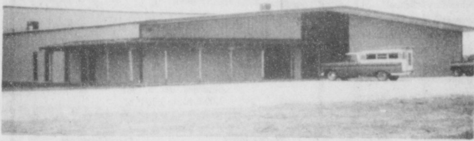
The new International Harvester building is now open on the Gruver Hiway---Drop by and see Dick Elbert and the gang---
