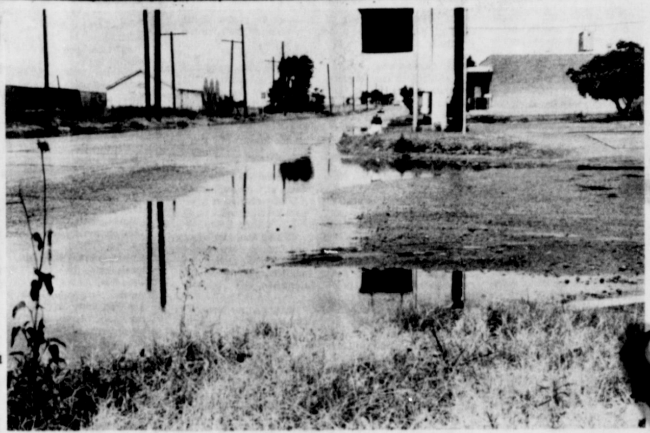
This accumulation of water on Interstate 40 at Commerce Street last Thursday is the way things also looked Wednesday after a slow, steady rain. For most of the week, there were many clouds but not much moisture, but the gray skies did give some relief from hot summer temperatures. (Staff Photo by Mike Haynes)
