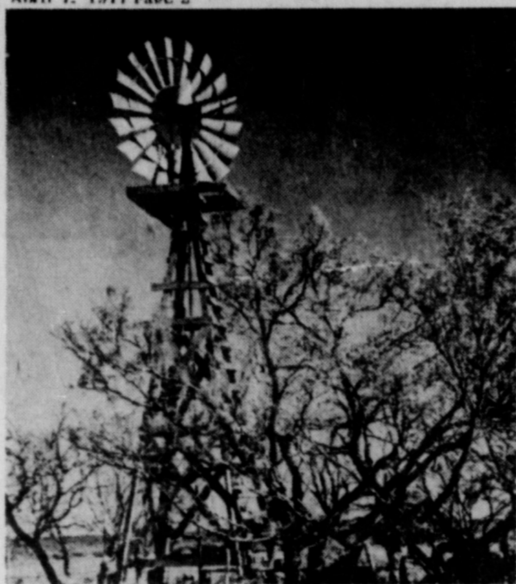
WINDMILLS FOR THE FUTURE —They may trigger memories of the past, but windmills are being considered as a source of power for the future, too. Agriculture Commissioner John C. White points out that harnessing wind power could supply the energy for such agricultural needs as pumping irrigation water and heating and cooling.
