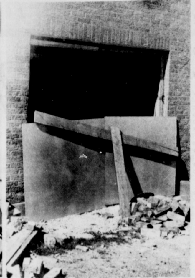
McLean High School is currently undergoing remodeling and repair. Above left, work has begun to lower ceilings and install air conditioning. Above right, a wall had to be removed in order for the boiler to be replaced. (Staff photos by Linda Haynes)
