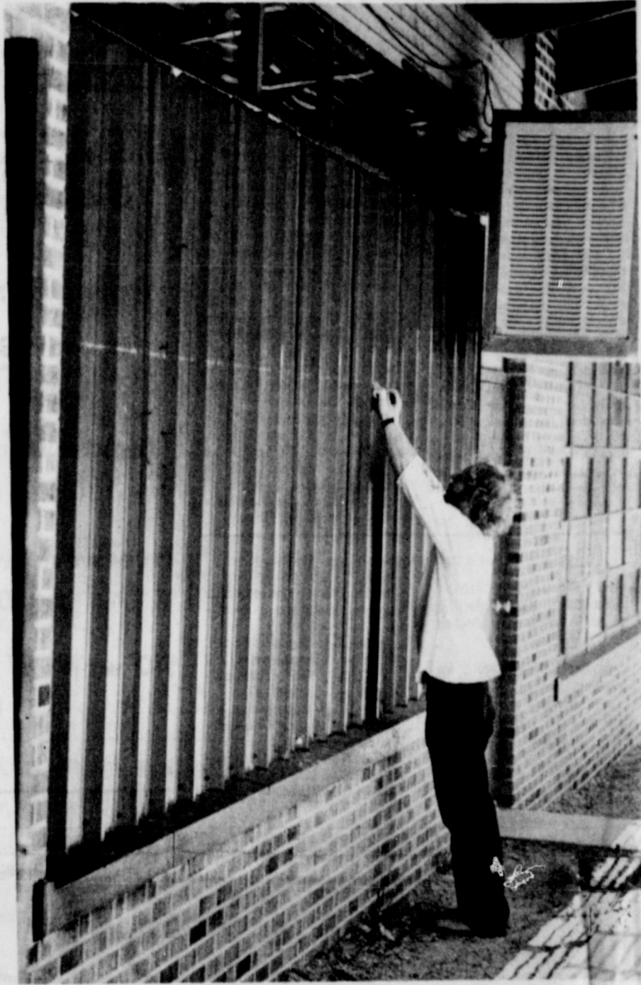
CUSTODIAN RON PRICE examines one of the new steel siding units at the McLean Elementary School. The unit pictured is one of three which has been installed at the school to cover window-walls, and help control heating and cooling. Superintendent Carl Dwyer said. The steel siding has 1 1/2 inches of insulation between the siding and the window, and then the inside is framed with 2 x 4's, padded with 3 1/2 inches insulation and covered with 5/8 inch sheetrock. Dwyer said that the school board will inspect the siding done by Arrowhead Industries of Amarillo at a cost of around $560 per unit before deciding whether to do the remaining 10 units in the building. (Photo by Linda Haynes)
