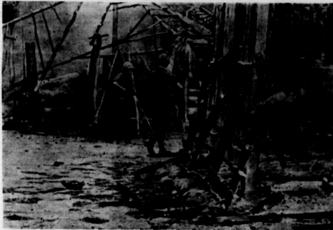
BURNING QUESTIONS—Soldiers of the First Infantry Division move carefully through the village of Tay Ninh in South Viet Nam, near the Cambodian border, after setting fire to suspected Viet Cong houses. Members of the division destroyed a major Viet Cong supply point here.
