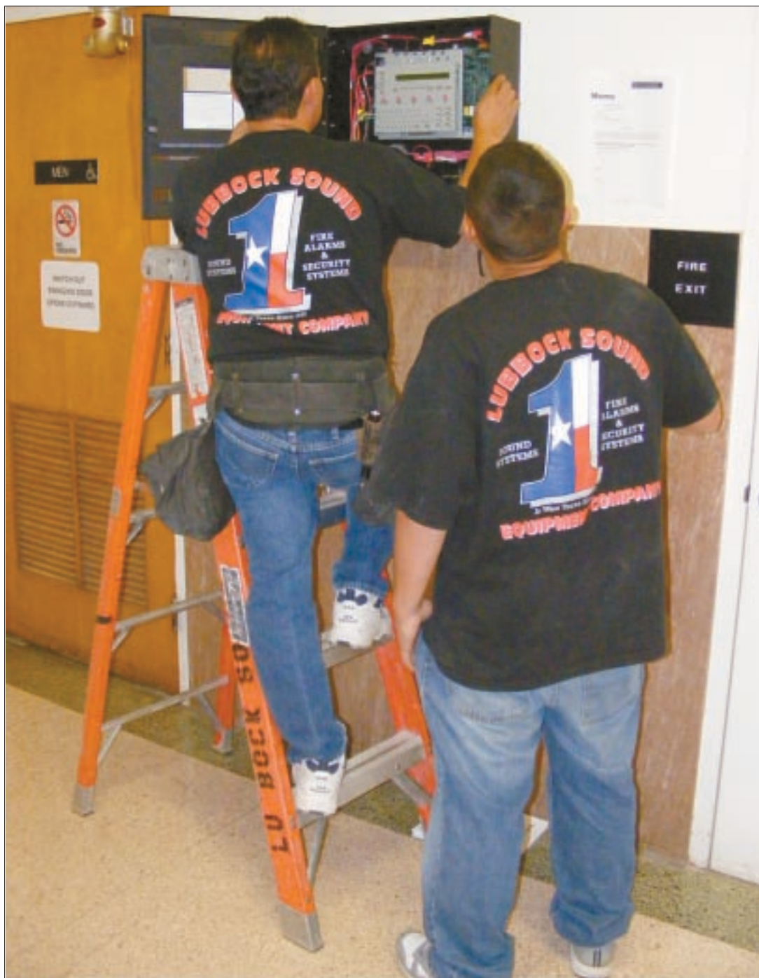
HERALD photo/Thomas Jenkins Technicians with Lubbock Sound and Alarm work on the fire alarm system at the Howard County Jail during a test of the system last week. According to county officials, the jail's new smoke evacuation system passed preliminary tests with flying colors. State jail commission inspectors will test the system Thursday.
